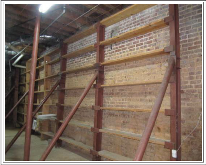
Basement Structure Reinforcement
