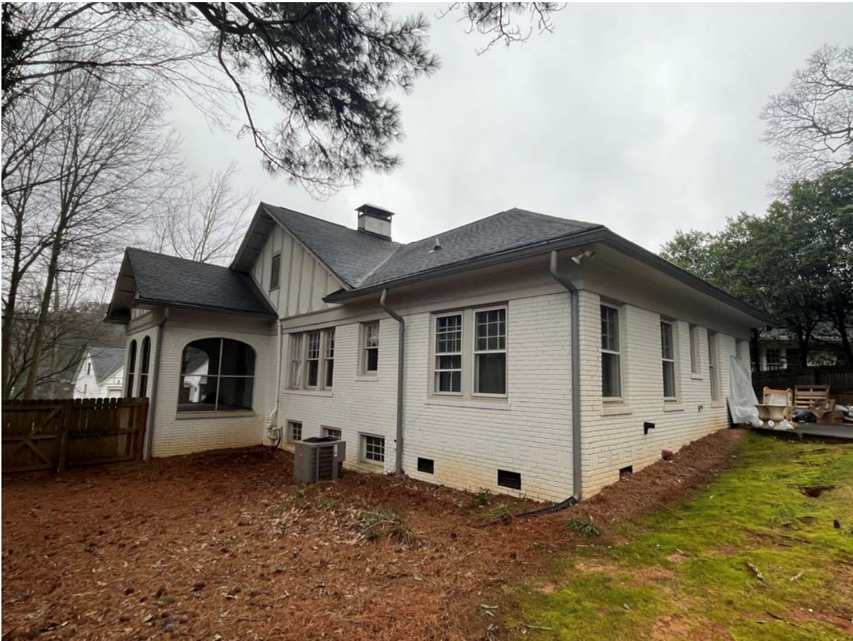
Right elevation from rear - area of addition
