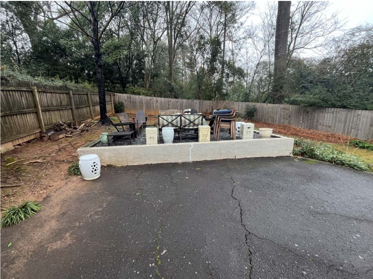
Existing gravel patio, block walls, and rear driveway to be removed
