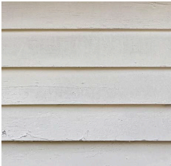
Siding Detail: Clapboard
