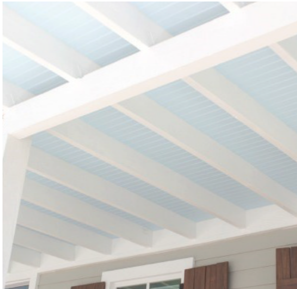
Ceiling finish: 4" nominal tongue and groove boards. Painted white (Greek Villa or similar)
