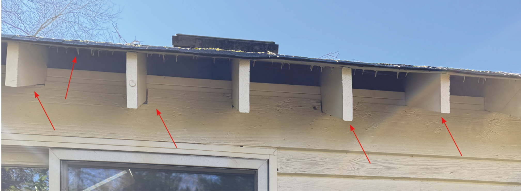
Re-roofed with 1in roofing nails on 1/4" sheathing. Miscellaneous, random joist sizing.
