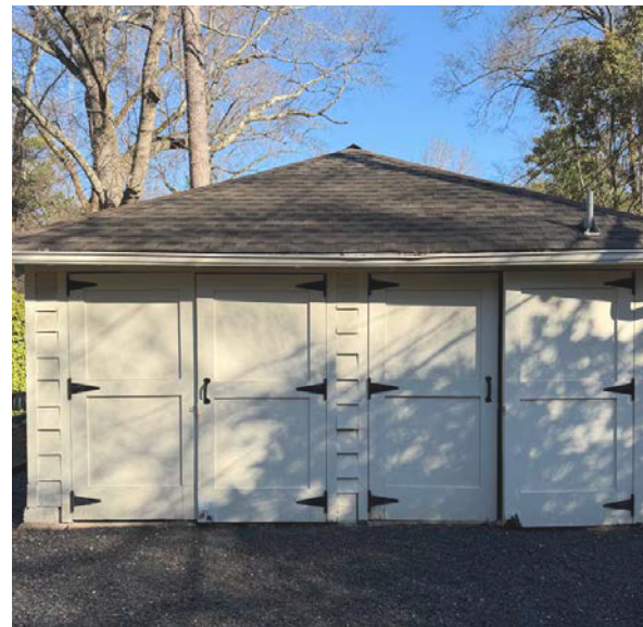
Roofing Geometry: Hip roof
