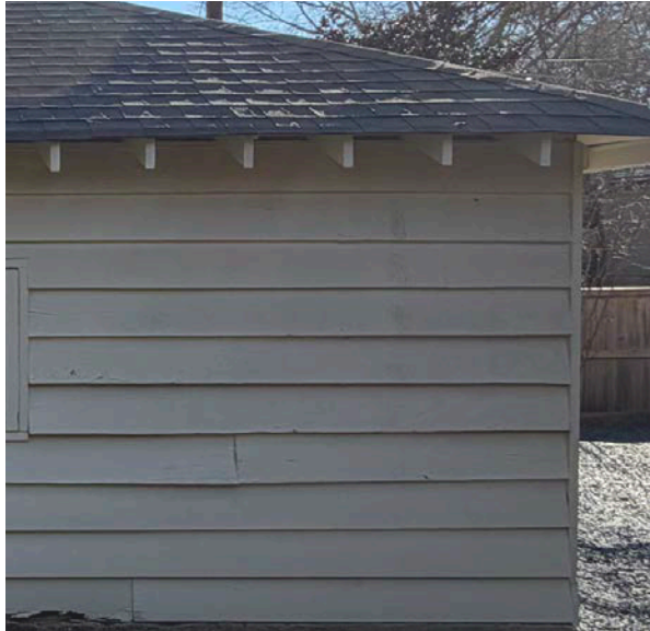
Roofing Detail: Open eaves
