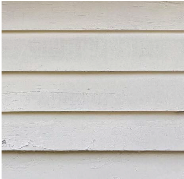
Clapboard wood siding: Color match existing and/or Sherwin Williams Greek Villa (to match existing)
