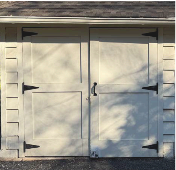
Doors: Carriage doors, two (2) pairs
