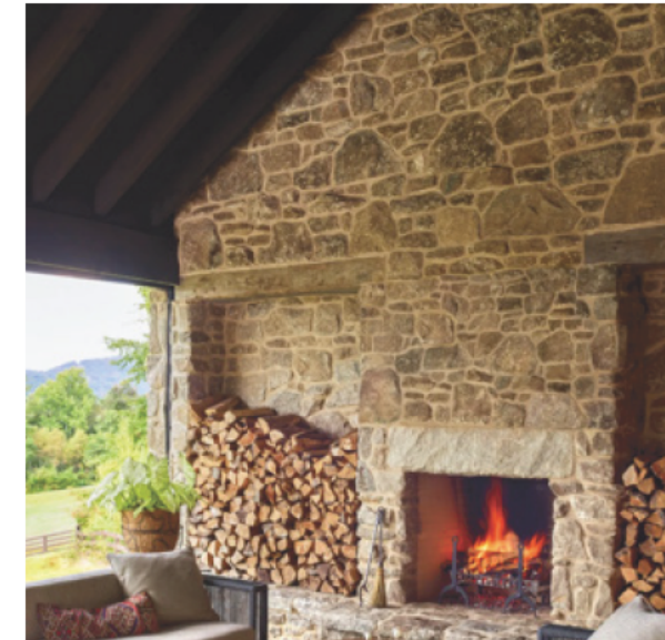
Stone chimney: Tan and light gray fieldstone with a mix of round and cut stone
