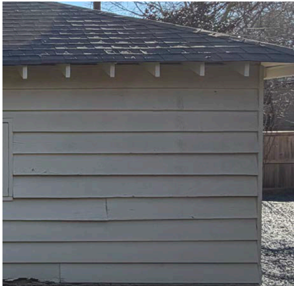
Roofing Detail: Open eaves
