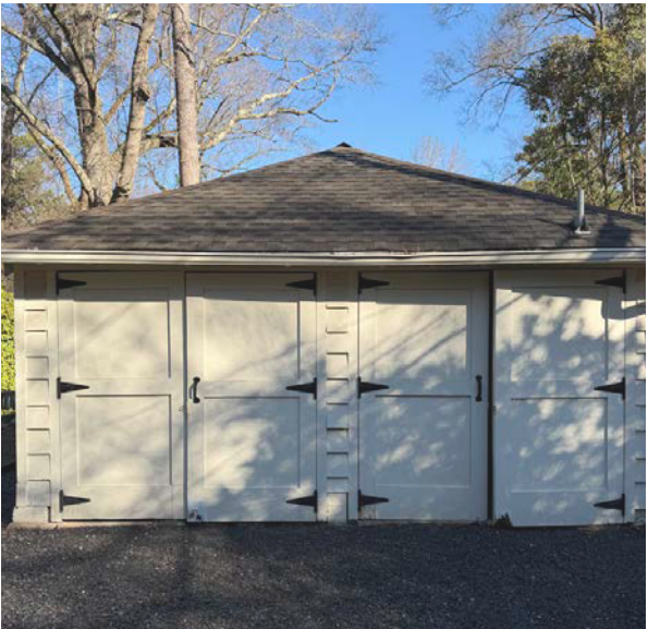
Roofing Geometry: Hip roof
