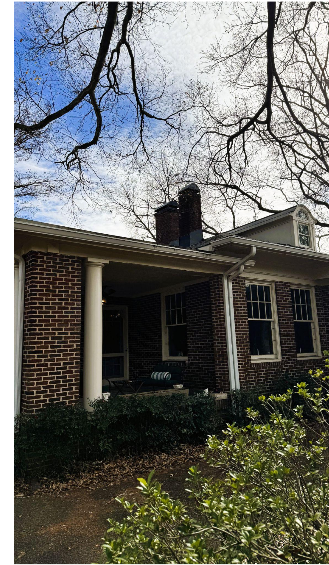
In the existing front porch and terrace the installation of railing is necessary for safety reasons and code regulations. The access to the porch has currently 5 steps and the downfall around this areas is greater than 36" to the ground, the homeowners expressed their concerns about it, and we proposed the installation of a typical iron wrought railing with minimal details to maintain the historic character of the property and comply with the modern code regulations
