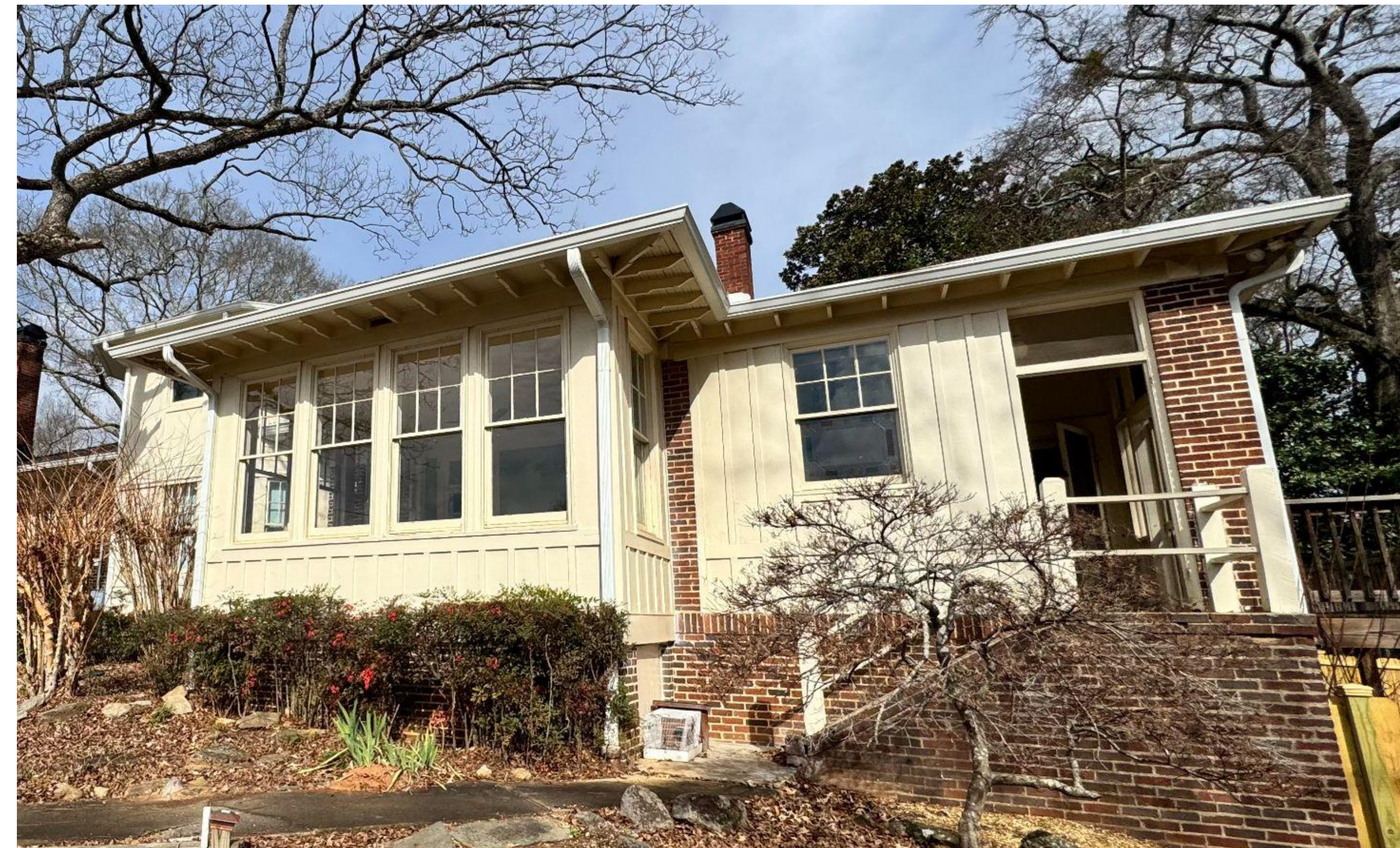
In this picture you can observe the architectural details to be repeated in the kitchen addition to create consistency in the new design: brick foundation, soldier brick course, board and batten, windows with 6 lites in top sash, roof overhang and rafters tail. Even the proposed rear access is consistent with original layout of window/ door location
