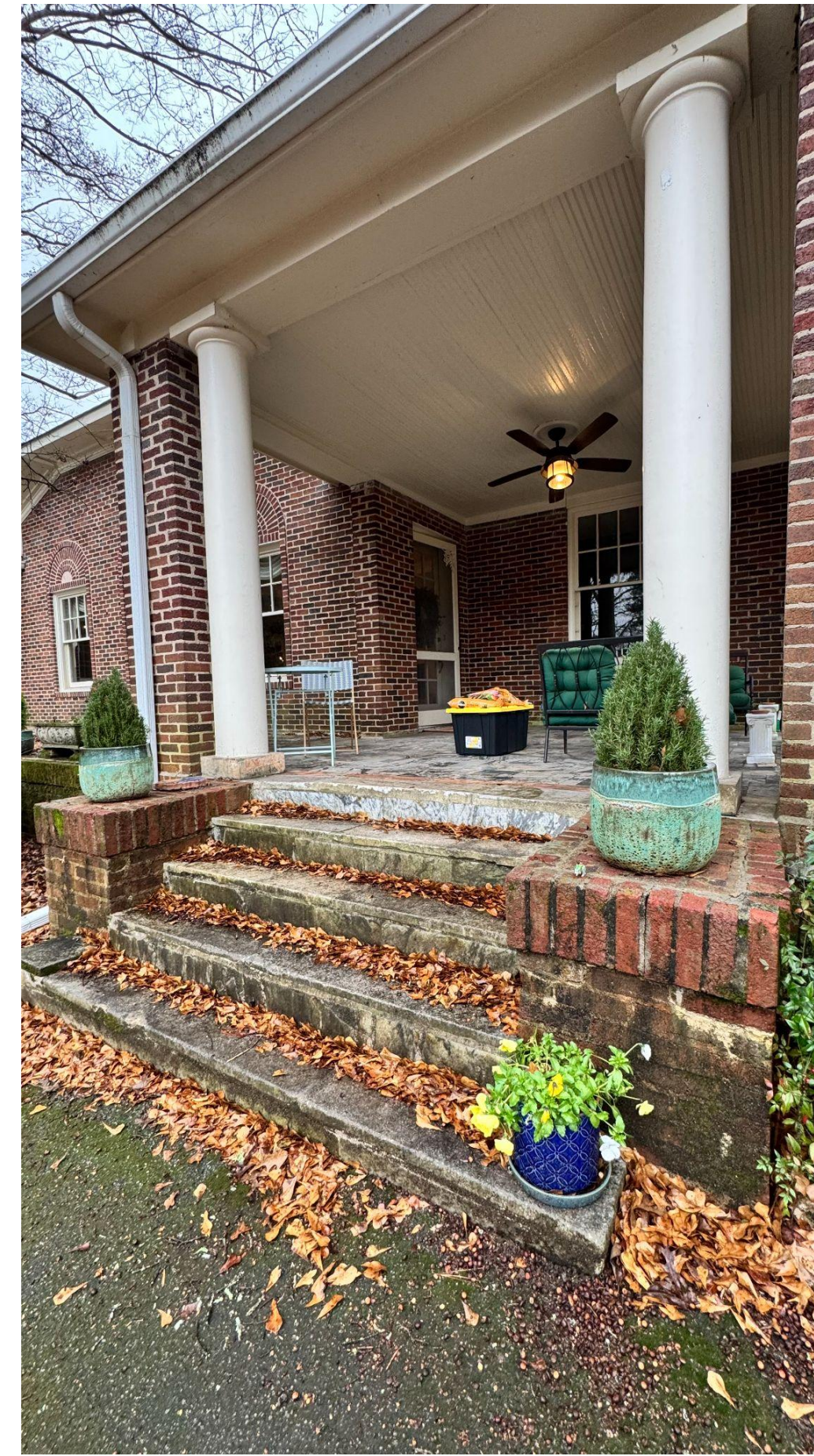
In the existing front porch and terrace the installation of railing is necessary for safety reasons and code regulations. The access to the porch has currently 5 steps and the downfall around this areas is greater than 36" to the ground, the homeowners expressed their concerns about it, and we proposed the installation of a typical iron wrought railing with minimal details to maintain the historic character of the property and comply with the modern code regulations
