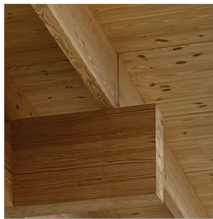
SOUTHERN YELLOW PINE RAFTERS & ROOF SOFFIT CLADDING
