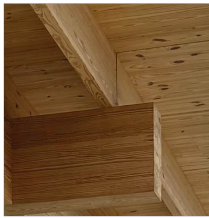
SOUTHERN YELLOW PINE RAFTERS & ROOF SOFFIT CLADDING
