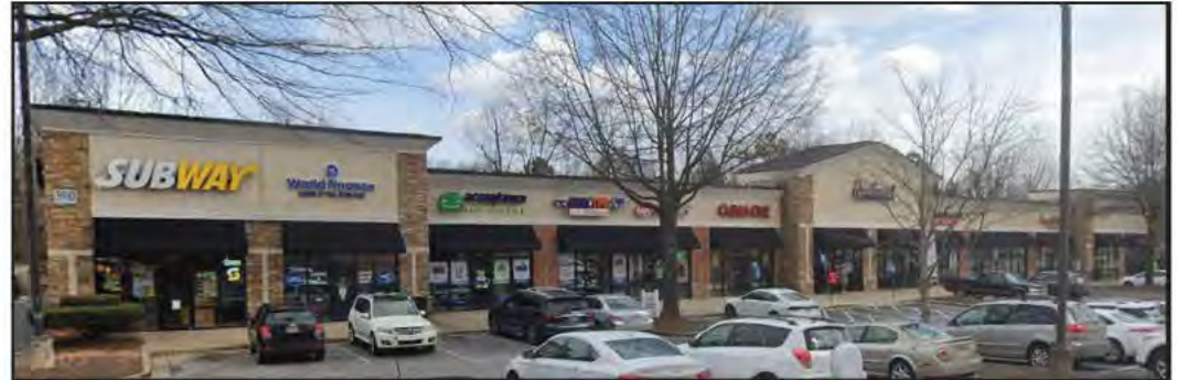
OVERALL VEIW OF FLAT SHOALS CROSSING
