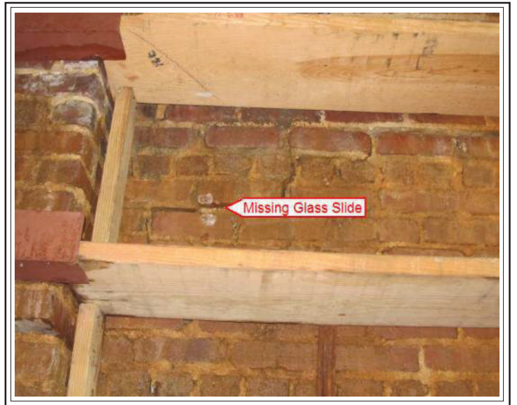
Basement Structure Reinforcement
