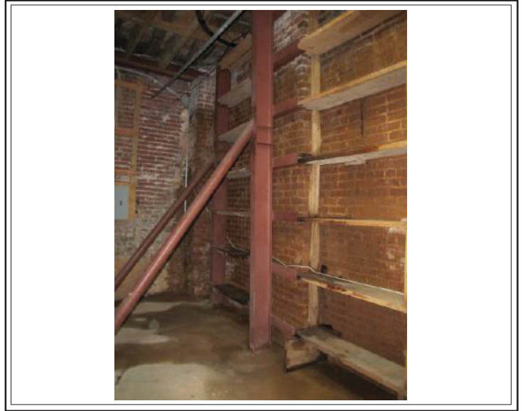
Basement Structure Reinforcement
