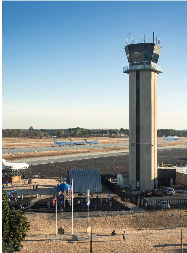
Figure 4-11: PDK Air Traffic Control Tower
