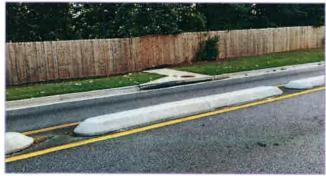
Figure 4: Median breaks allow stormwater to drain while reducing water velocity
