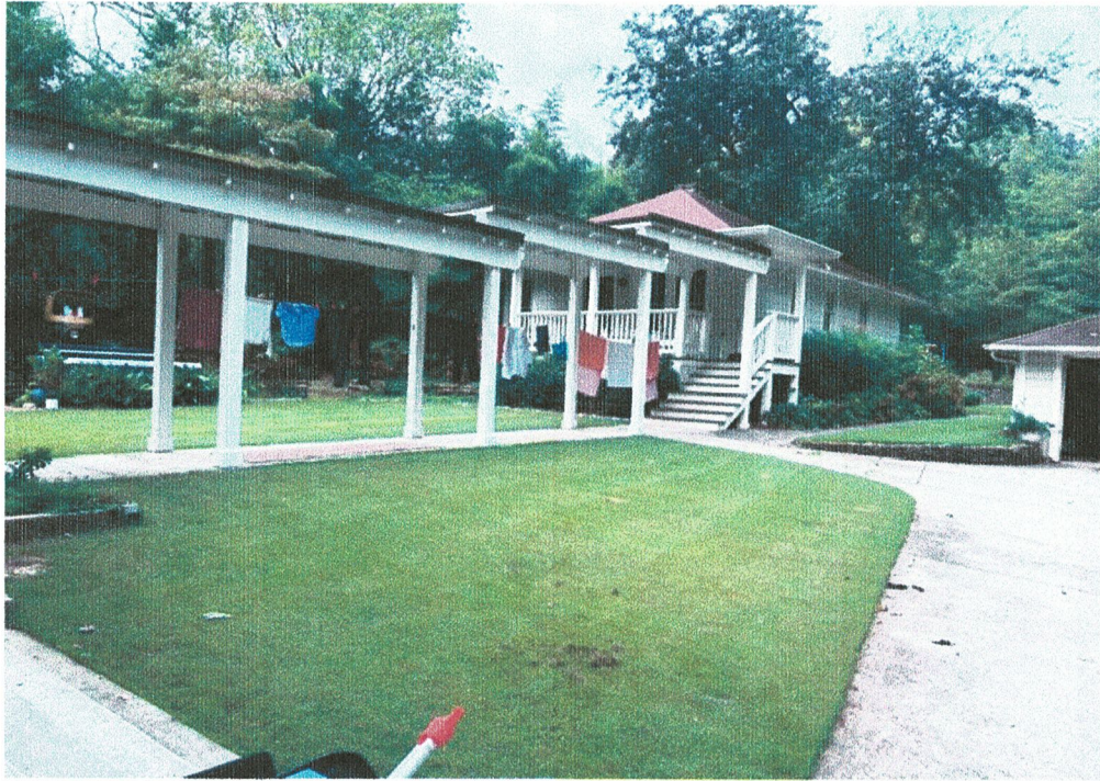
Approach from driveway
