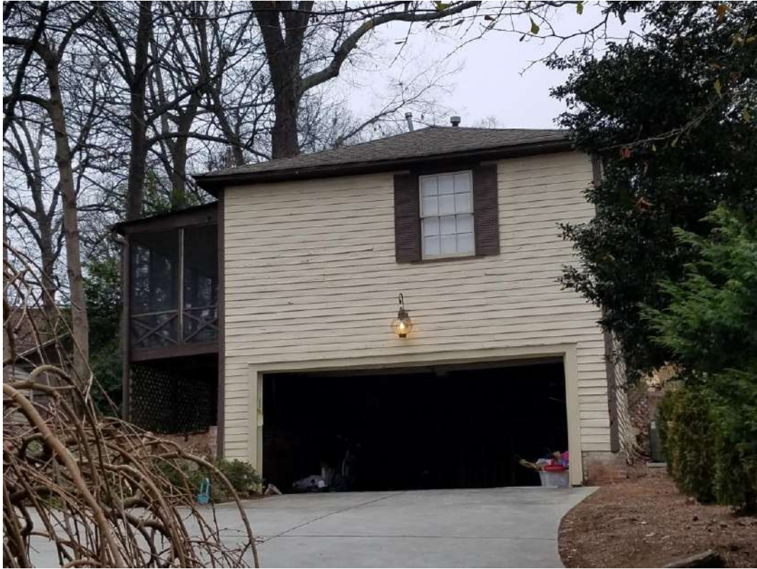
Front garage wall. New footings and portal framed header required.
