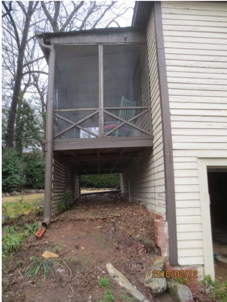
Side porch to be re-built
