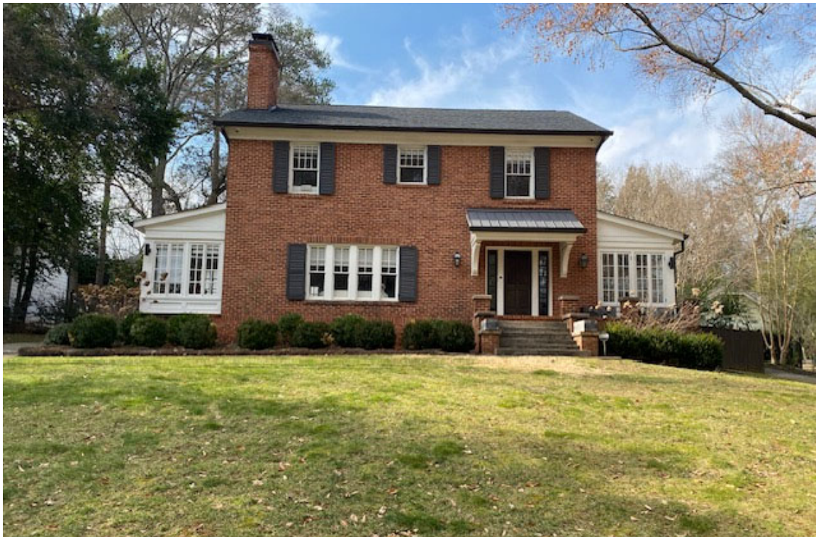
View of Front Elevation from Street
