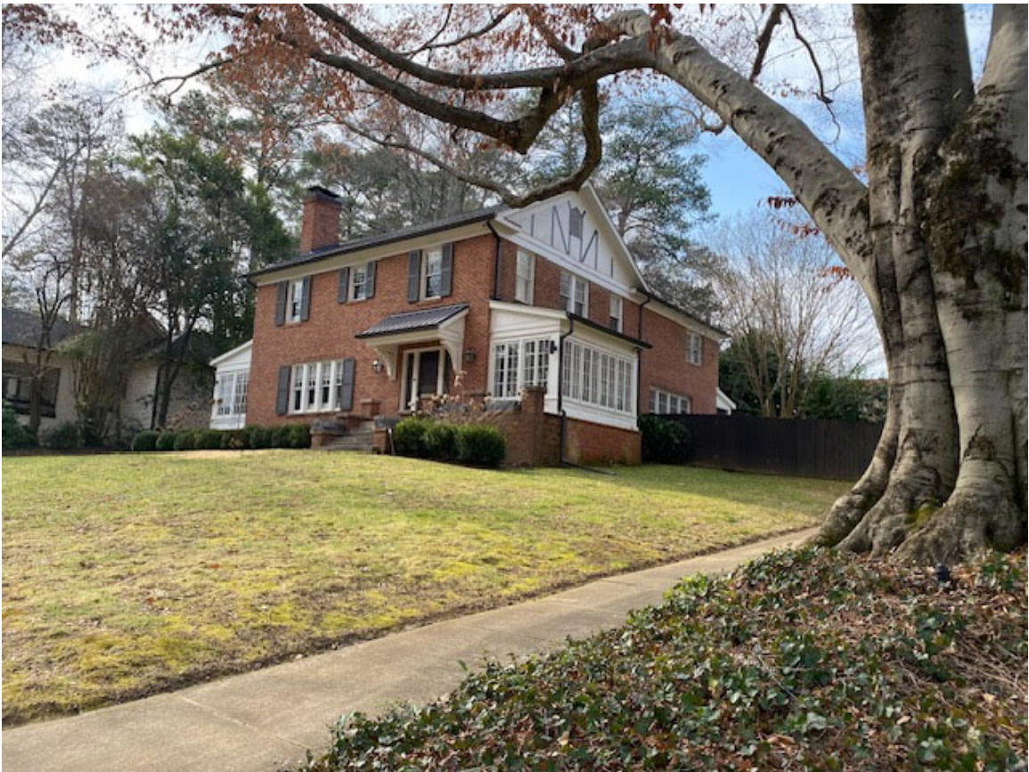
View from Right side R.O.W.
