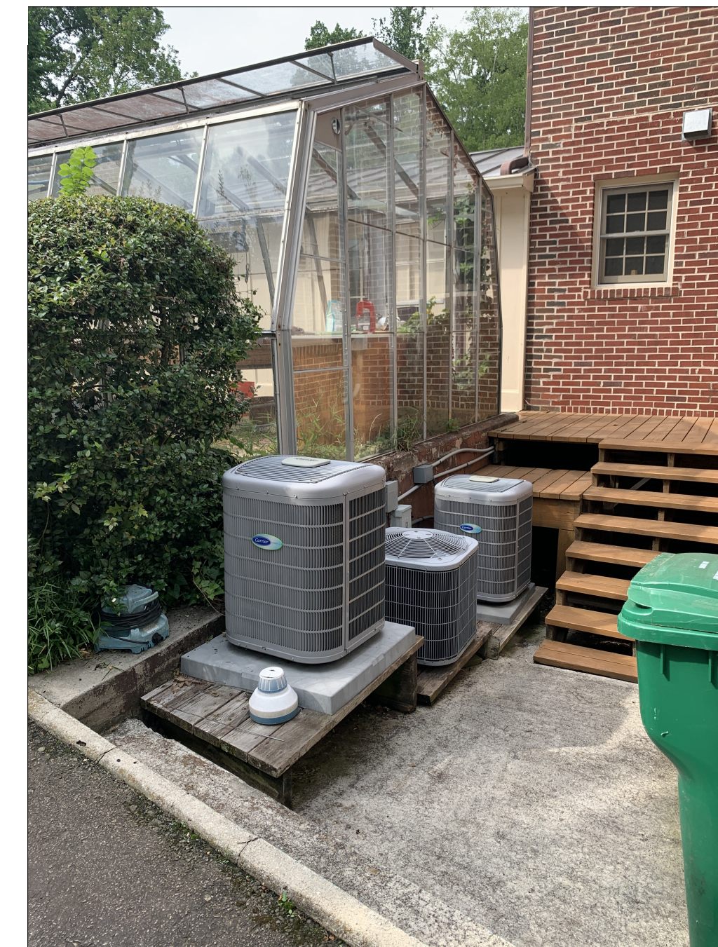
CONCRETE LANDING AT REAR
