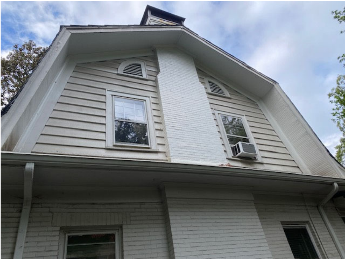
View of Side Gambrel Roof Gable (facing driveway)
