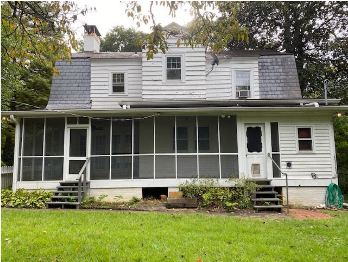
View of Rear Elevation
