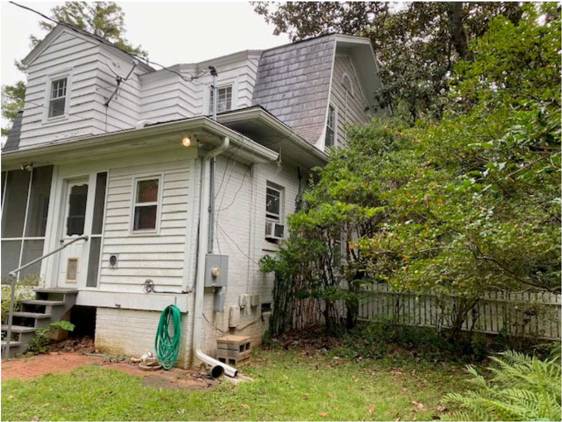
View from Rear Yard (location of Main Level BR Addition)
