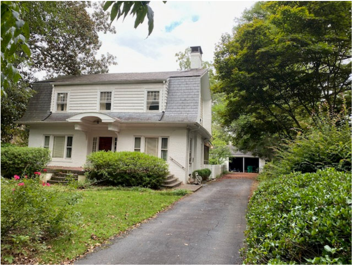
View from Right side R.O.W.
