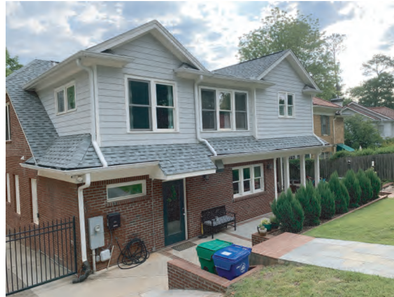
Existing rear facade of the home. The carriage house will have shed dormers with siding and the lower level of the carriage house will be brick to match the existing house as closely as possible.
