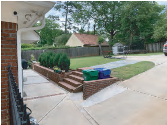
View of existing rear concrete patio. The wall and stair are to be reconfigured as shown on the proposed site plan and permeable paving to be placed where the concrete is, in order to meet the lot coverage allowance. This is to be reviewed by the ZBA for zoning compliance.
