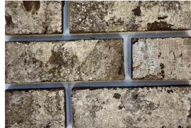
Brick infill to match existing
