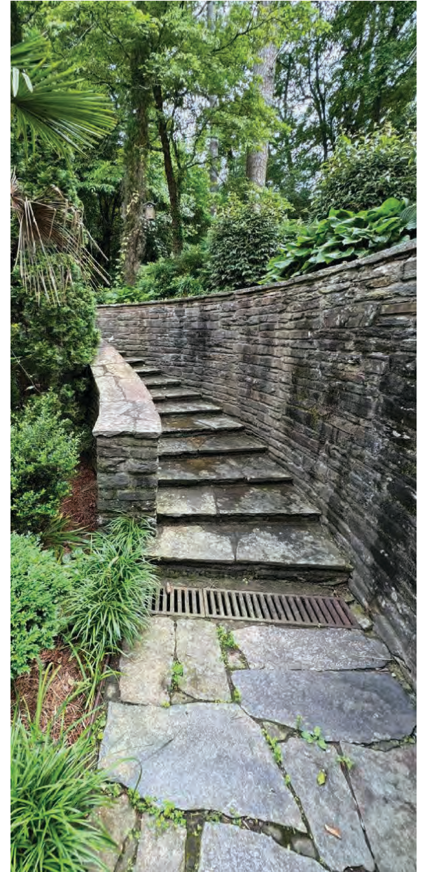
EXISTING STONE STEPS
