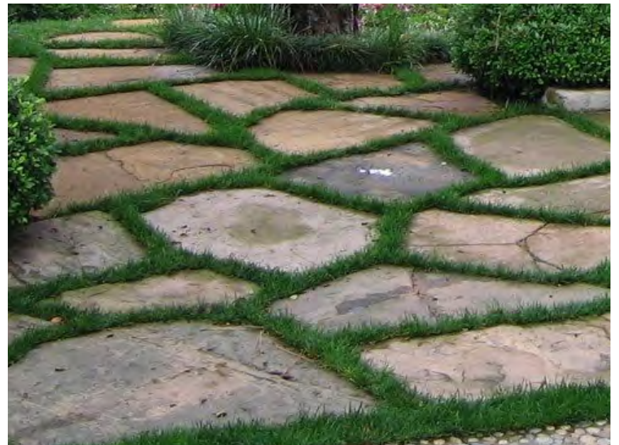
IRREGULAR STONES WITH PLANTED JOINTS
