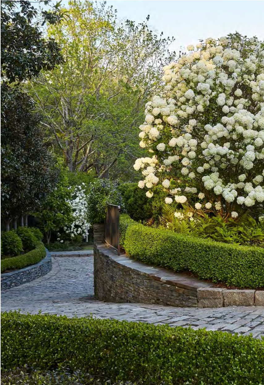
STACKED STONE RETAINING WALL
