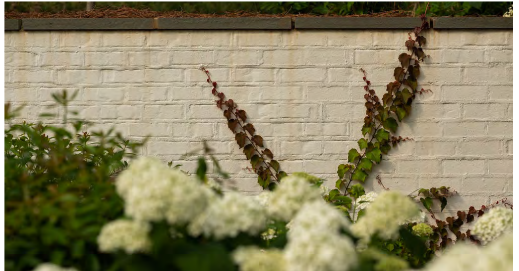
PAINTED BRICK WALL WITH STONE CAP
