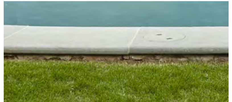
ELEVATED POOL COPING
