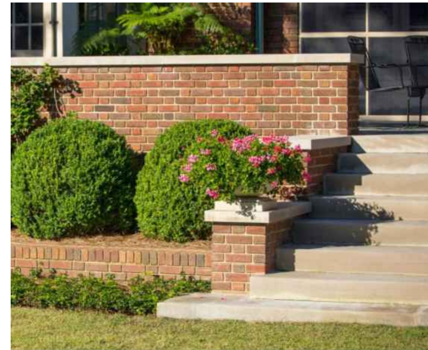
BRICK WALL WITH LIMESTONE CAP
