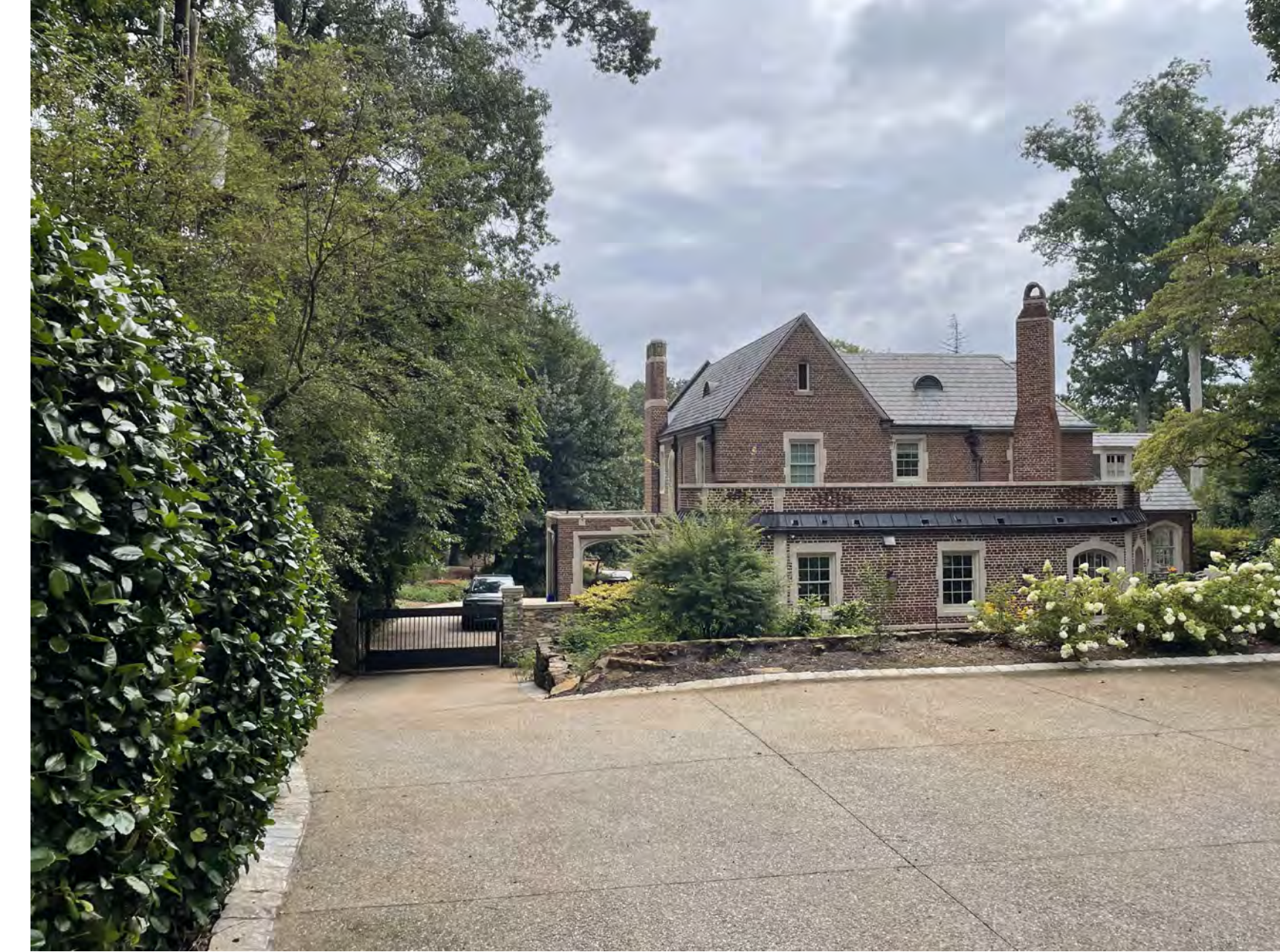
REAR AND WEST HOUSE FACADE
