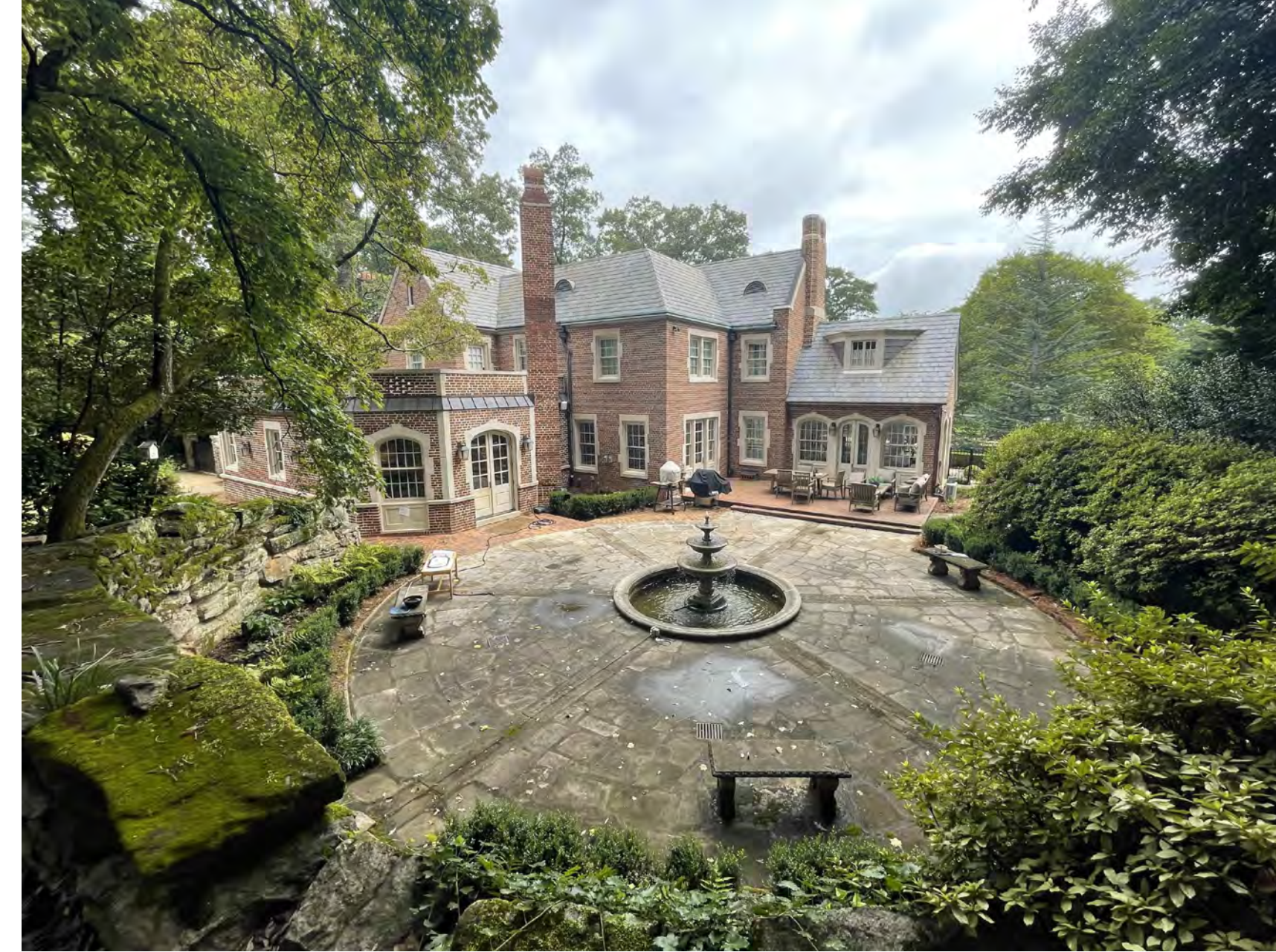
REAR AND EAST HOUSE FACADE
