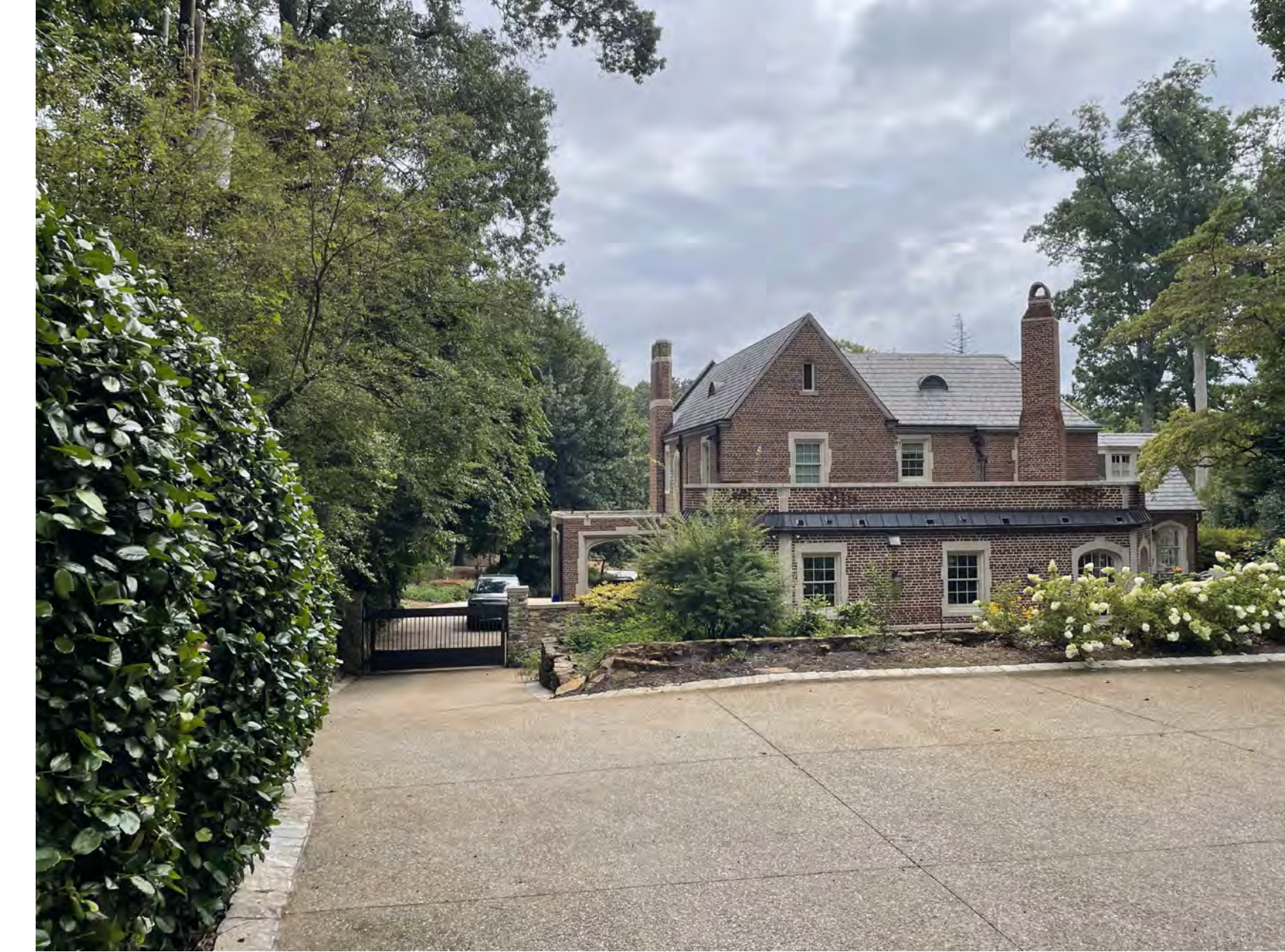
REAR AND WEST HOUSE FACADE
