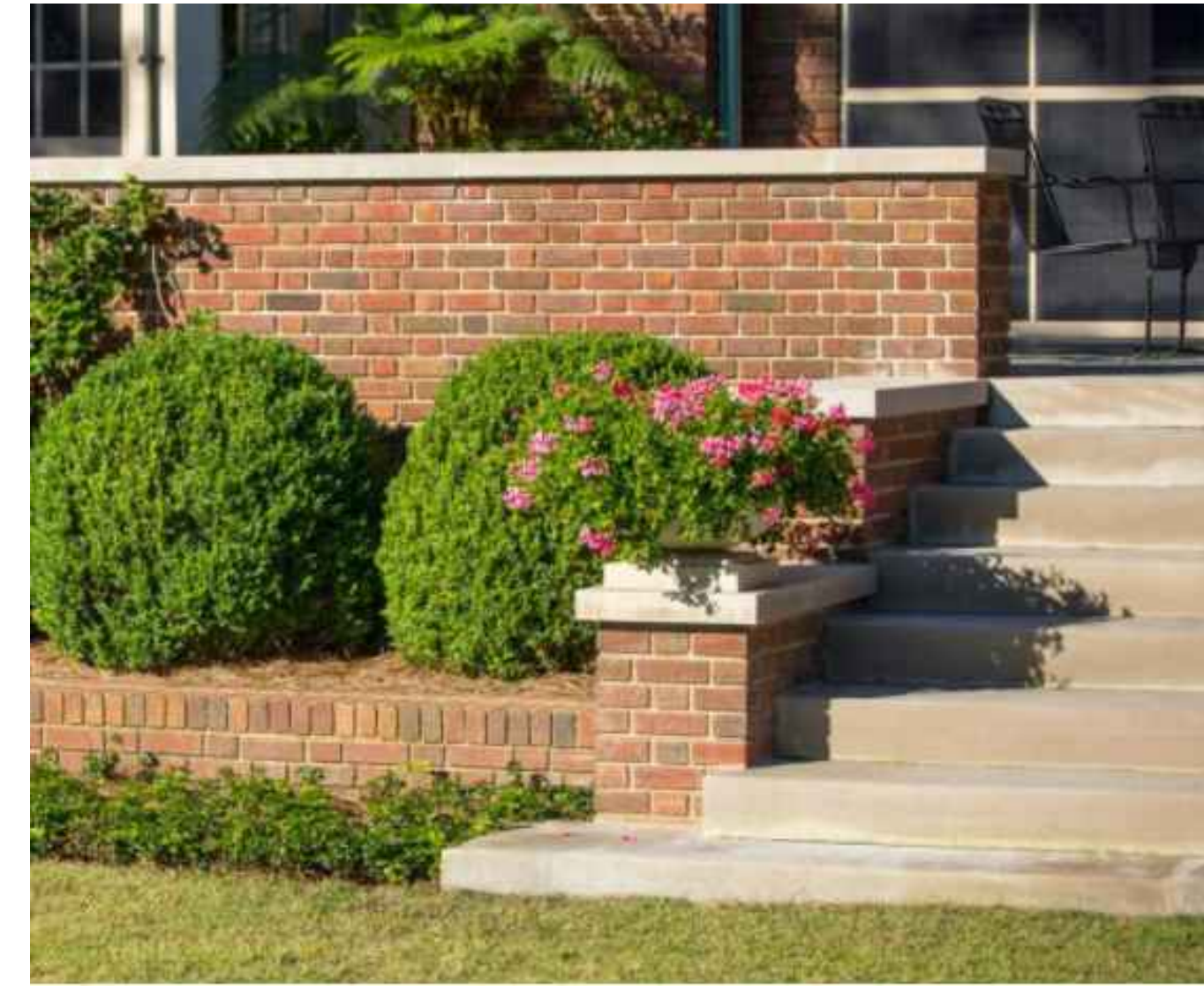
BRICK WALL WITH LIMESTONE CAP
