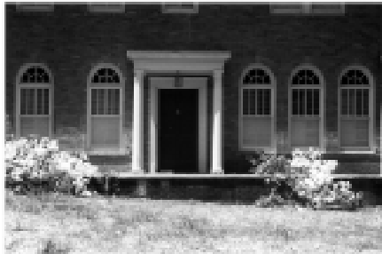
This group of round arched windows is a characteristic feature of the Italian Renaissance Revival style.
