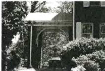
THE OPEN CHARACTER OF THIS PORTE COCHERE IS AN IMPORTANT FEATURE THAT SHOULD BE RETAINED
