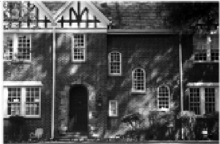
The row of stepped windows on this house provides the front facade with a distinctive pattern that should be maintained.
