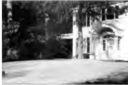
Entire front yard space has been graveled to provide parking; front yard landscape lost
