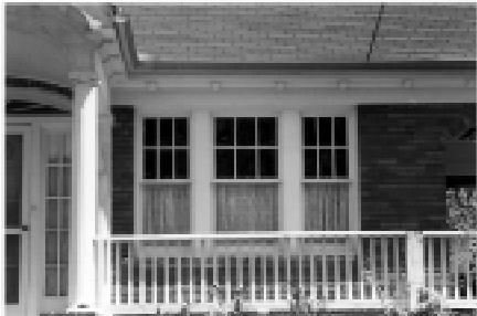
These double-hung windows, with six-over-one pane configuration typical of the Craftsman style, have been well-maintained.
