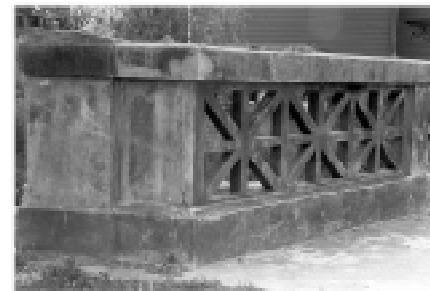
View of architecturally significant bridge balustrade over Peavine Creek at Oxford
