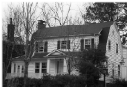
Typical Dutch Colonial Revival House with side-gabled gambrel roof and front shed dormer.
