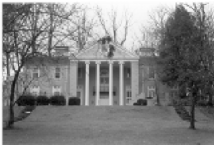
Example of portico with square masonry corner columns.
