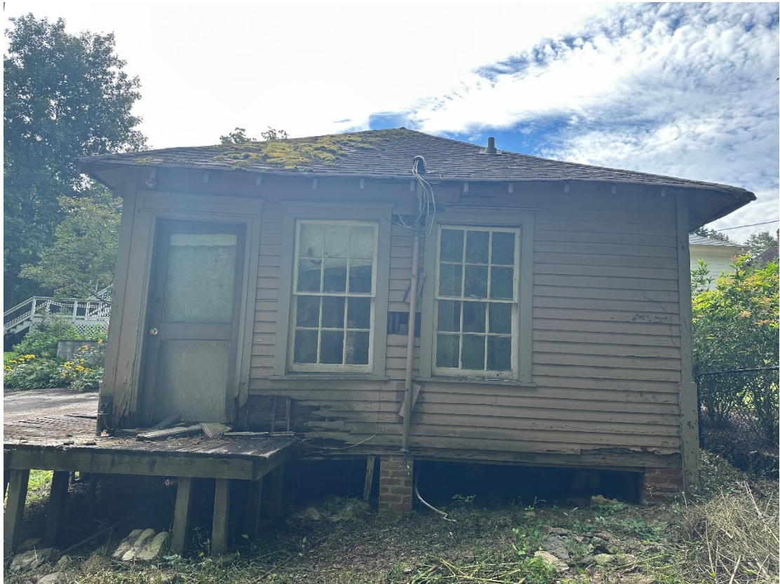
Above: right-hand (northwest) side of carriage house
