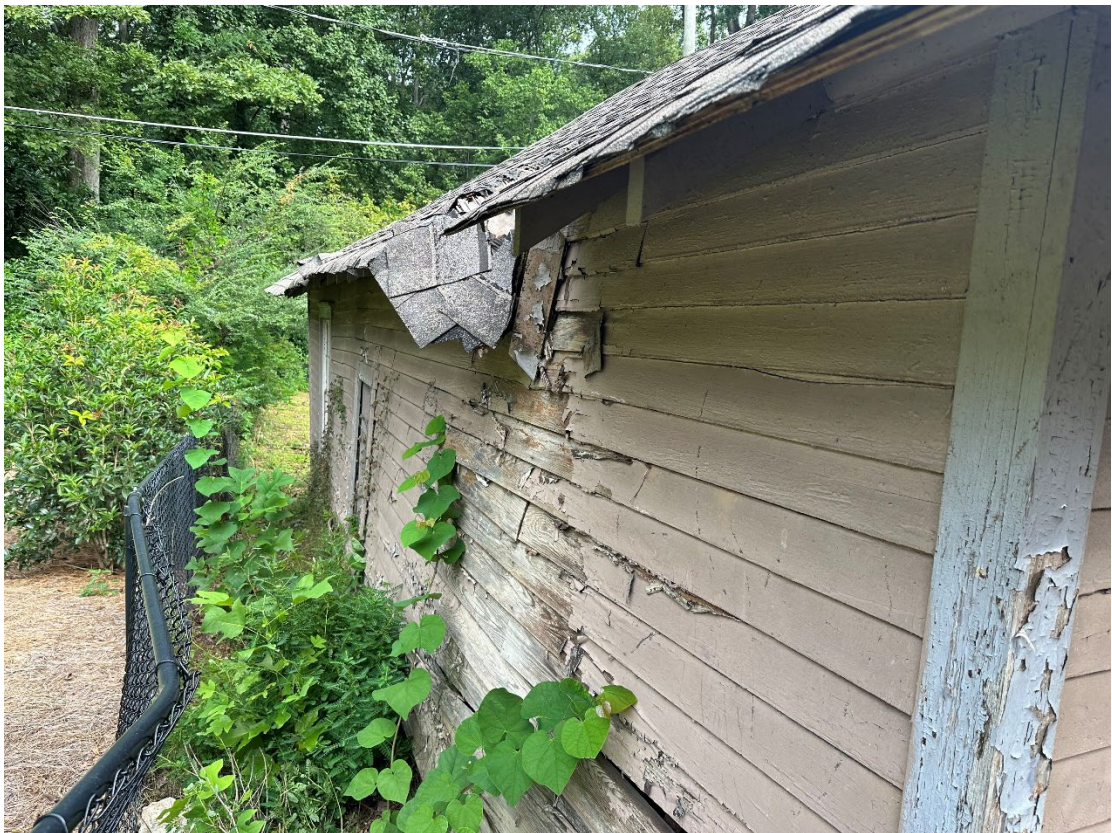
Above: Rear (southwest side) of carriage house
