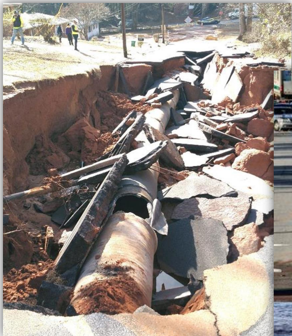
Celia Way January 2023 Prestressed Concrete July 08, 2024
