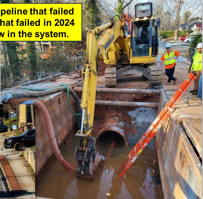
McLendon Road 42" diameter Feb/April 2024 Prestressed Concrete
