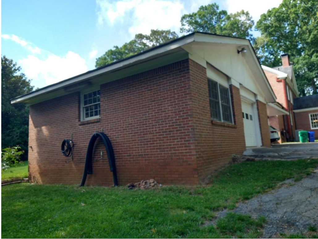
Existing Garage North elevation
