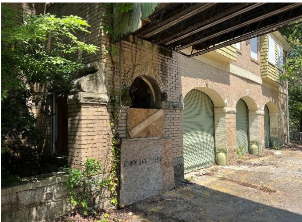
IMG CH1-3: Connection point between bridge from Solarium to second floor. Previous entry below now boarded up.
