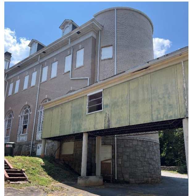
IMG EX2-4: Closer look at the Solarium half circle stair addition as well as the addition of the bridge that connects to the Carriage House.
