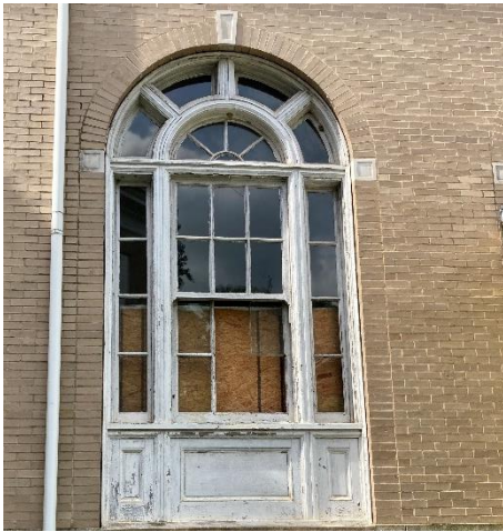
IMG EX5-1: Typical arched window lining the Solarium.
