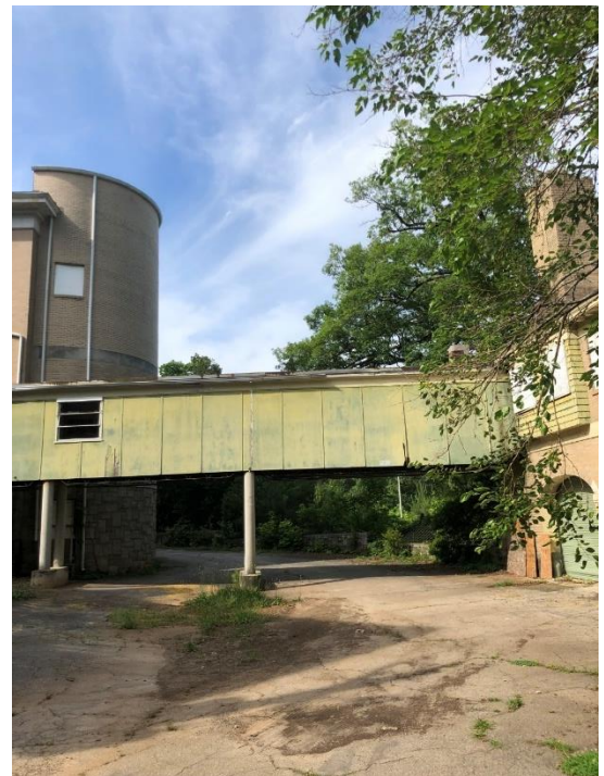
IMG CH1-5: Bridge connection from Main House to Carriage House which is to be demolished.
