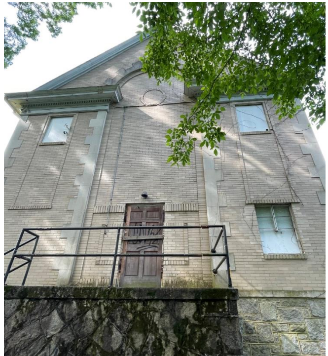
IMG EX1-4: Organ Room addition along with Music Room behind.
