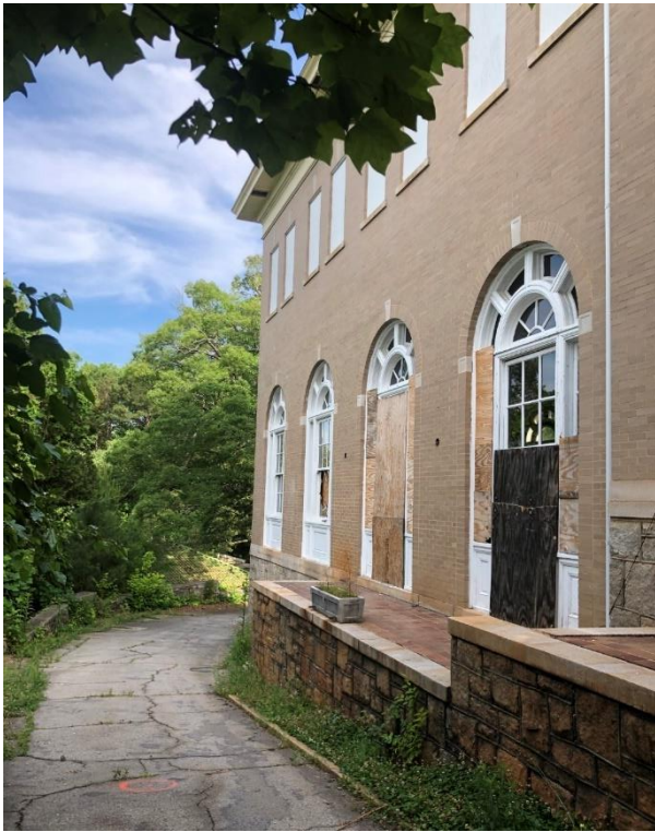
IMG EX3-1: Southeast view of the arched windows only present in the Solarium. Door will be inserted onto closest window per ADA requirements.
