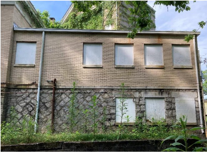
IMG EX1-1: Northeast portion of the Candler Mansion outside of the service kitchen. Overgrowth in the back.
