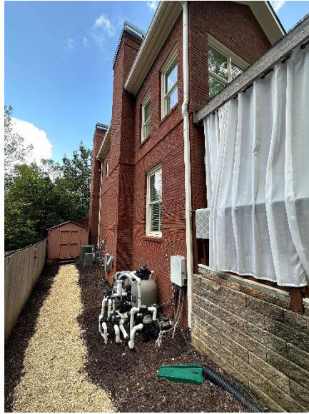
Photo 3 – View of West Side of 1141 Empire As Seen From Rear Yard of Property
