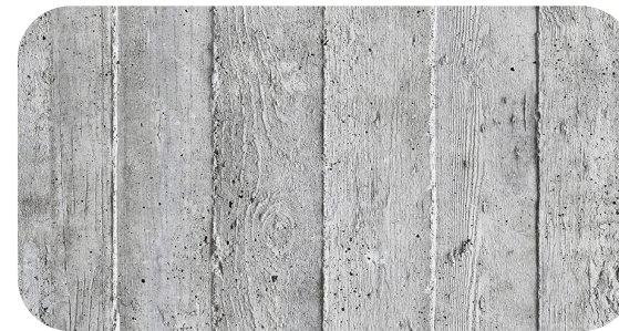
BOARD-FORM CONCRETE Exposed Foundation
