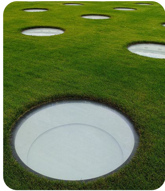
SKYLIGHTS Toddler Playground
