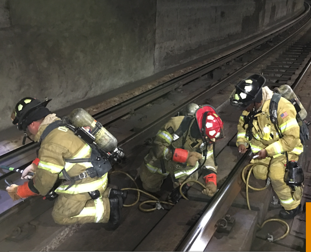
Crew working to bypass high powered electrical rail through a technique called shunting.
