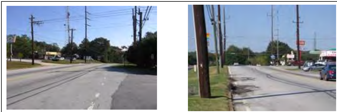
Overhead power lines
