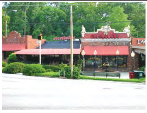
Utility consolidation at Emory village, Atlanta
