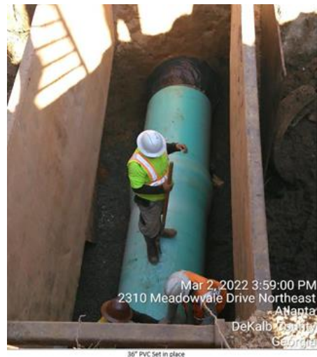
Cityworks Document 03-02-22 2225 Heritage Drive Pipe Replacement - Evidence of debris; evidence of repairs
